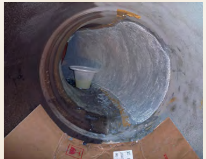
Application of Loctite® Nordbak® Pneu Wear.
