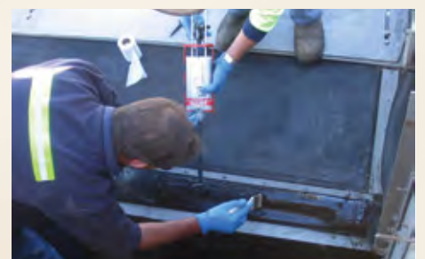
Rebuilding the decant gate hinge with Loctite® Fixmaster® Rapid Rubber Repair
