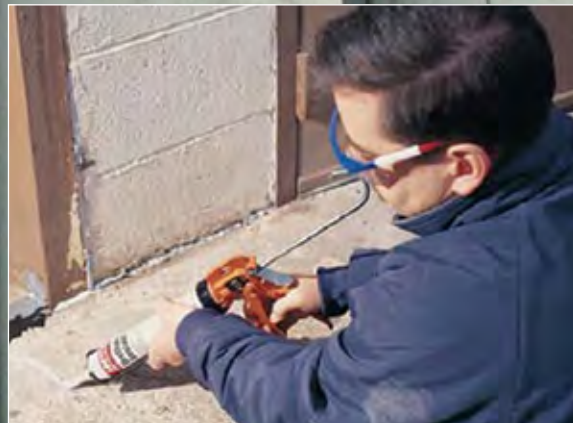
Filling concrete cracks with Fixmaster® Urethane Sealant
