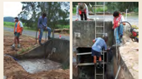
Re-surfacing the culvert walls with Magna-Crete saved over 7 weeks labour
