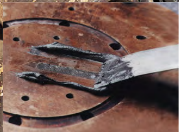
Repairing mechanical damage with Fixmaster® Steel Putty
